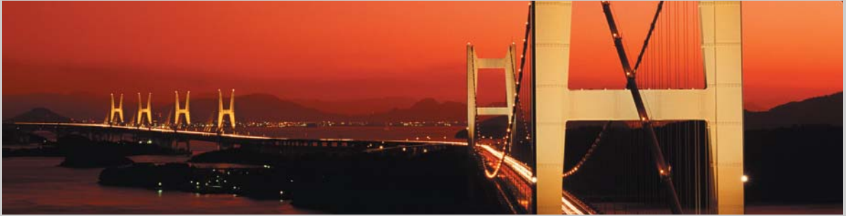
Japan's Seto Ohashi Bridge
